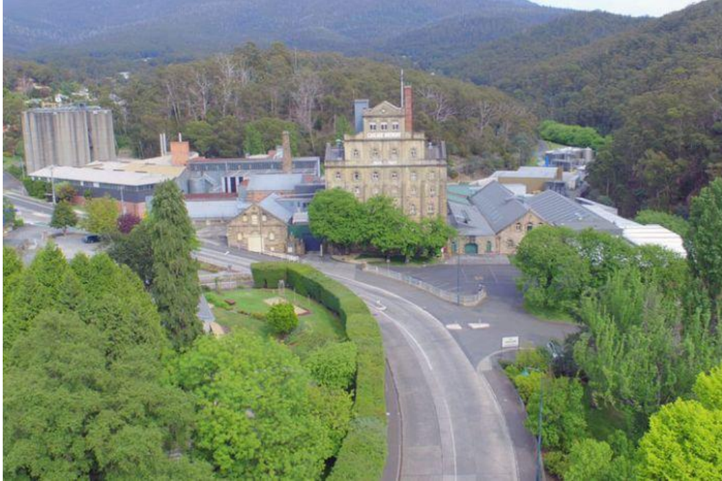
Before the cable car development (Supplied)
